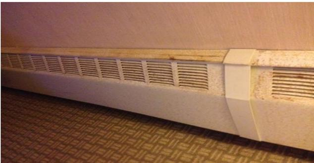
Hot air spreads out, becoming less dense and rising in the air. This creates a vacuum, pulling cool air towards the baseboard heater and starting the process over again. A natural convection process takes place as cold air enters the bottom of the element, is heated and then lifted as it comes in contact with the hot element and released back into the room. While baseboard heating is inexpensive to install, it has several drawbacks.
